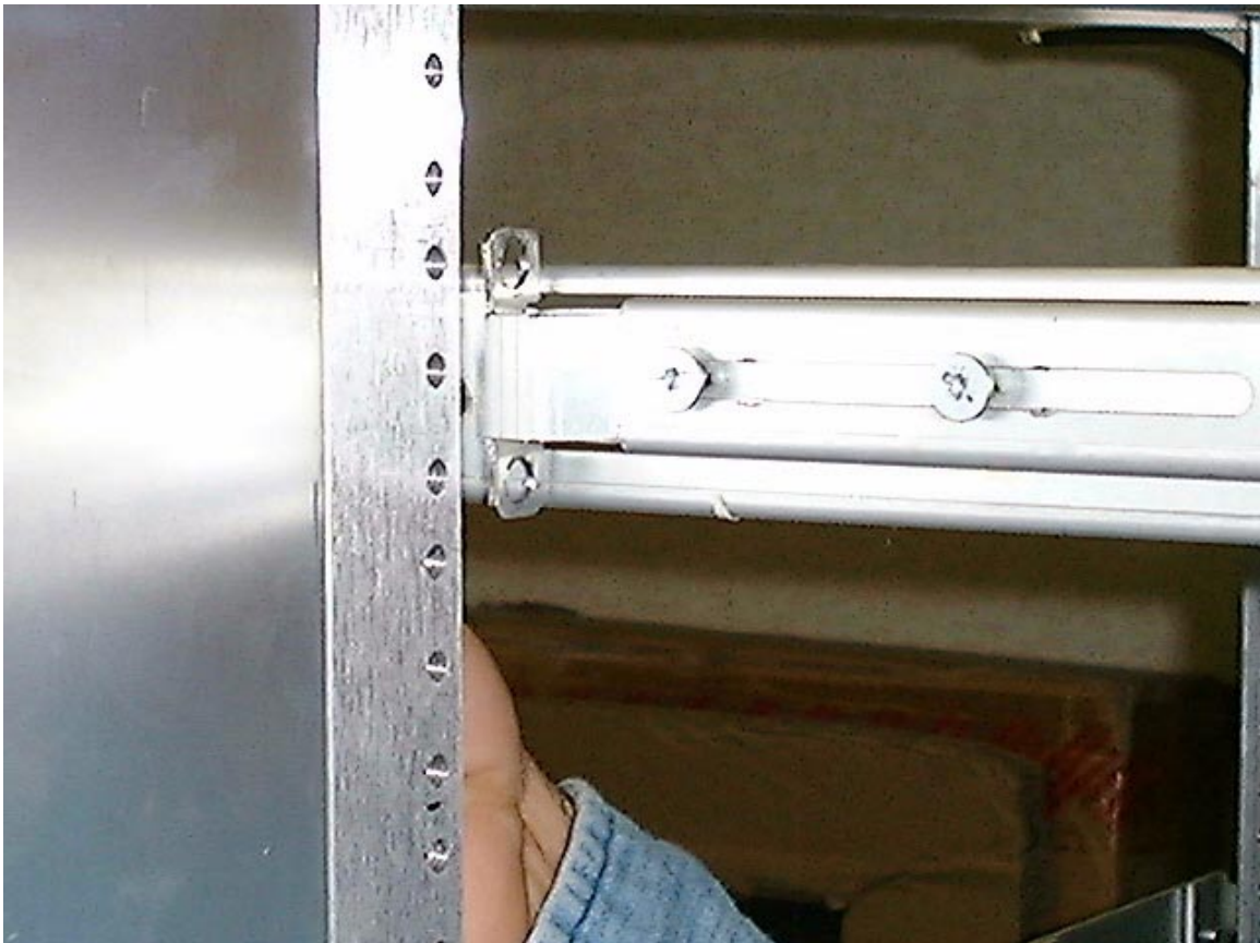
Figure 7: Bracket mount adjustment screws on the Compaq Telco Rack Option Kit rack rails
